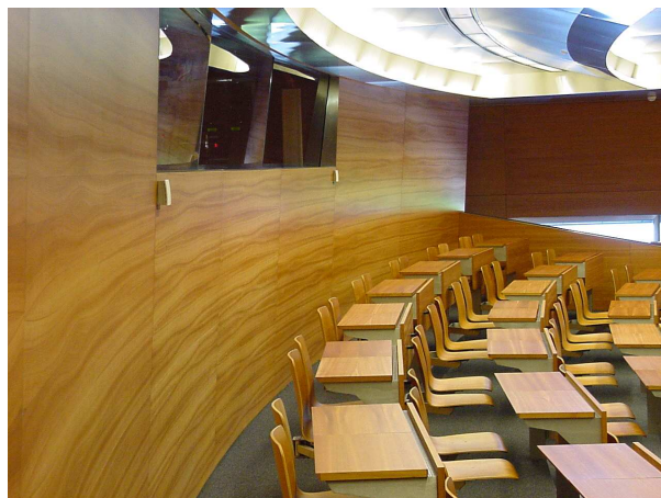
Figure 3: Rear wall of a lecture hall (not the same room as in figure 1), which throws an annoying echo back toward the front area, with or without the sound system.
